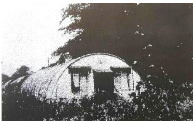
A 1950 picture of one of the former Llanover Park camp huts which was converted into a residence.
