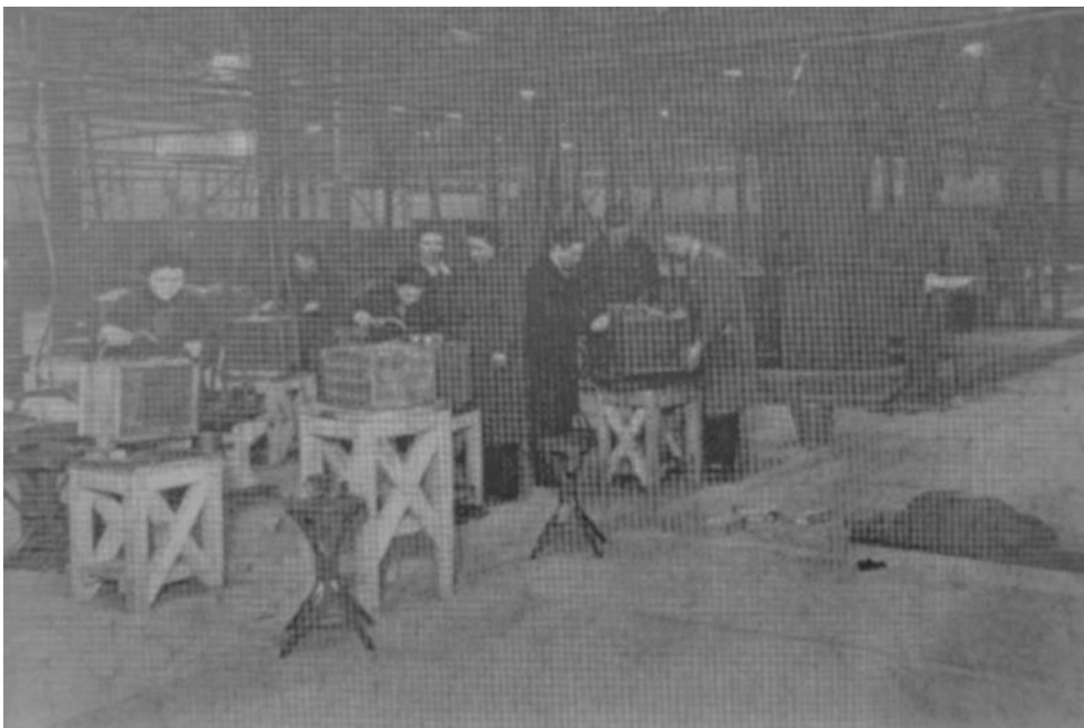
The first of the few. Finishing off the first of the radiators.
