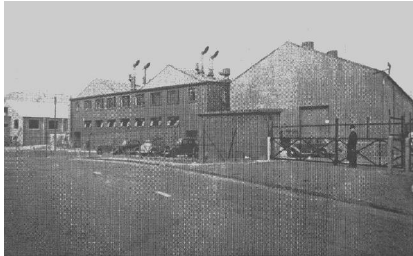
Front view of Llanfoist Works showing new offices in the foreground.
